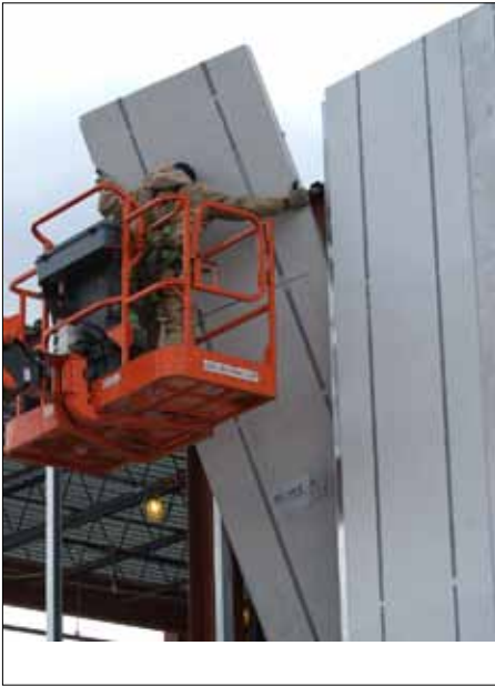
ACCEL-E wall panels frame, insulate and sheath in one easy step.
